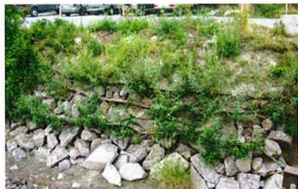
Typical riprap with vegetated soil wrap
