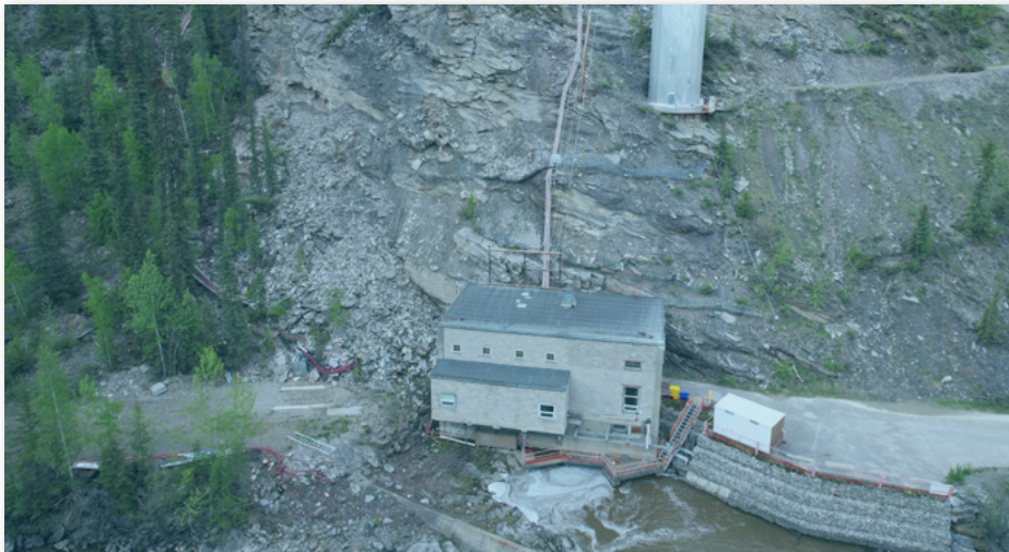
Mayo A hydro facility is impacted by erosion, leading to ground instability. Dangerous slope conditions make it difficult to access the plant for regular maintenance or operational emergencies.
