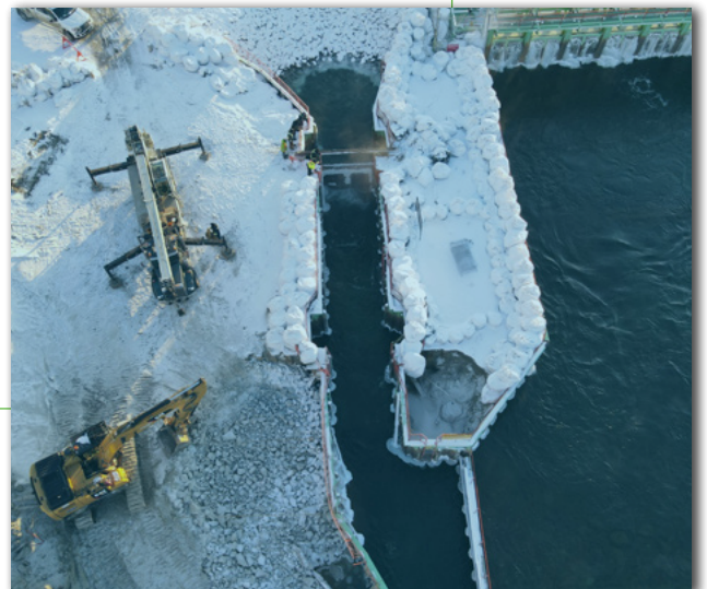
Repairing the Lewes River boat lock
