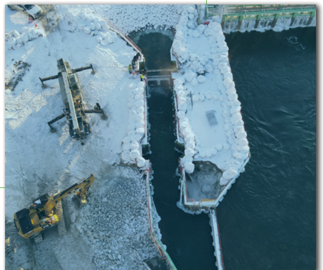
Repairing the Lewes River boat lock
