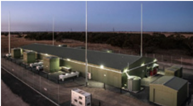
30 MW/8 MWh battery in South Australia Photo credit: ARENA
