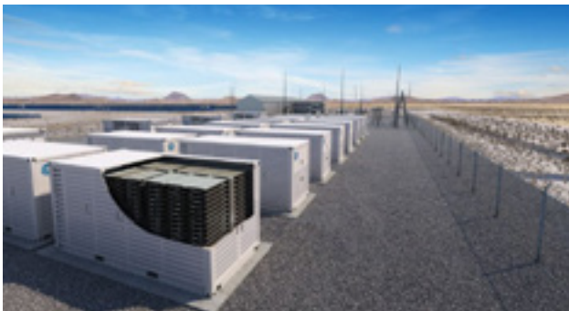
Modular battery installation Photo credit: GreenTech Media
