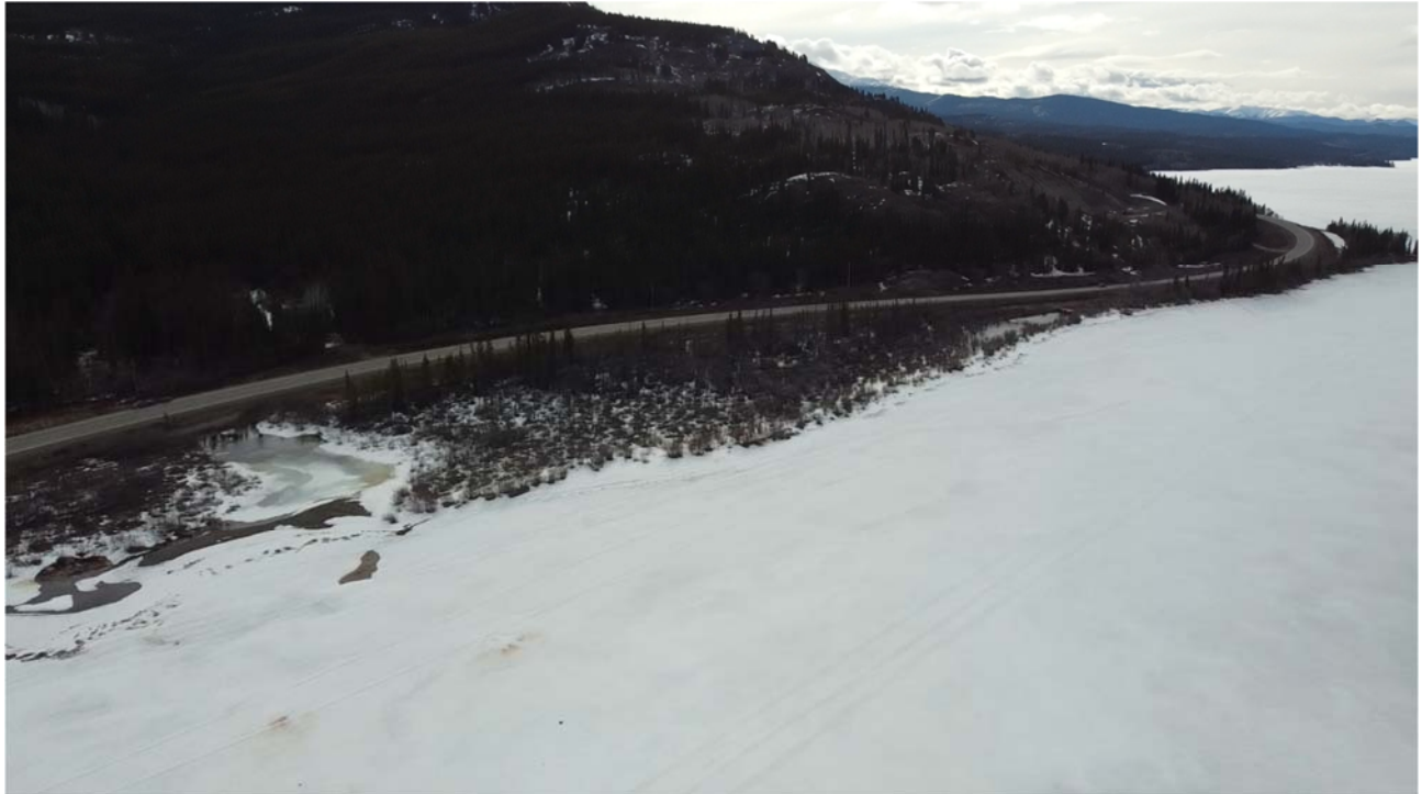
Photo 9. View of conditions at monitoring site ML1 (unnamed creek mouth on Marsh Lake) on May 4, 2022.
