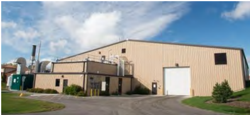
Figure 12 Oshkosh garage-style biogas plant
