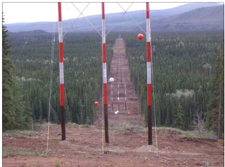
At Stewart River looking south. Photo: Yukon Energy
