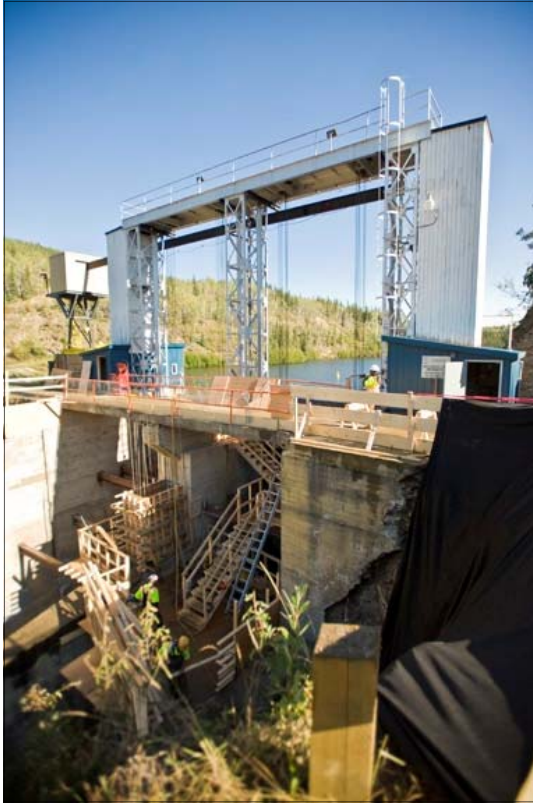
Construction on the Wareham Lake dam. Photo: Archbould.com
