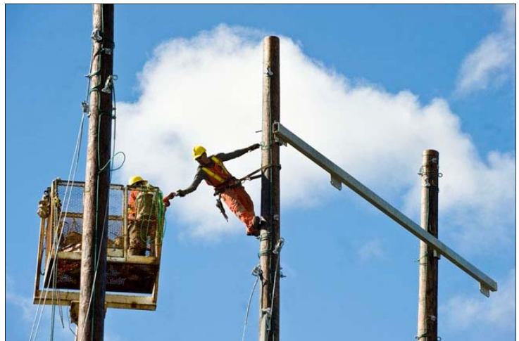
Installing crossbars. Photo: www.archbould.com
