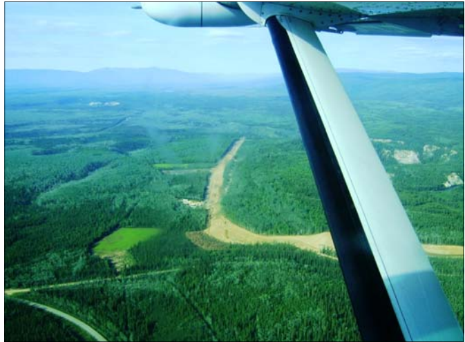
Aerial view of cleared penstock route to the Mayo B powerhouse.
