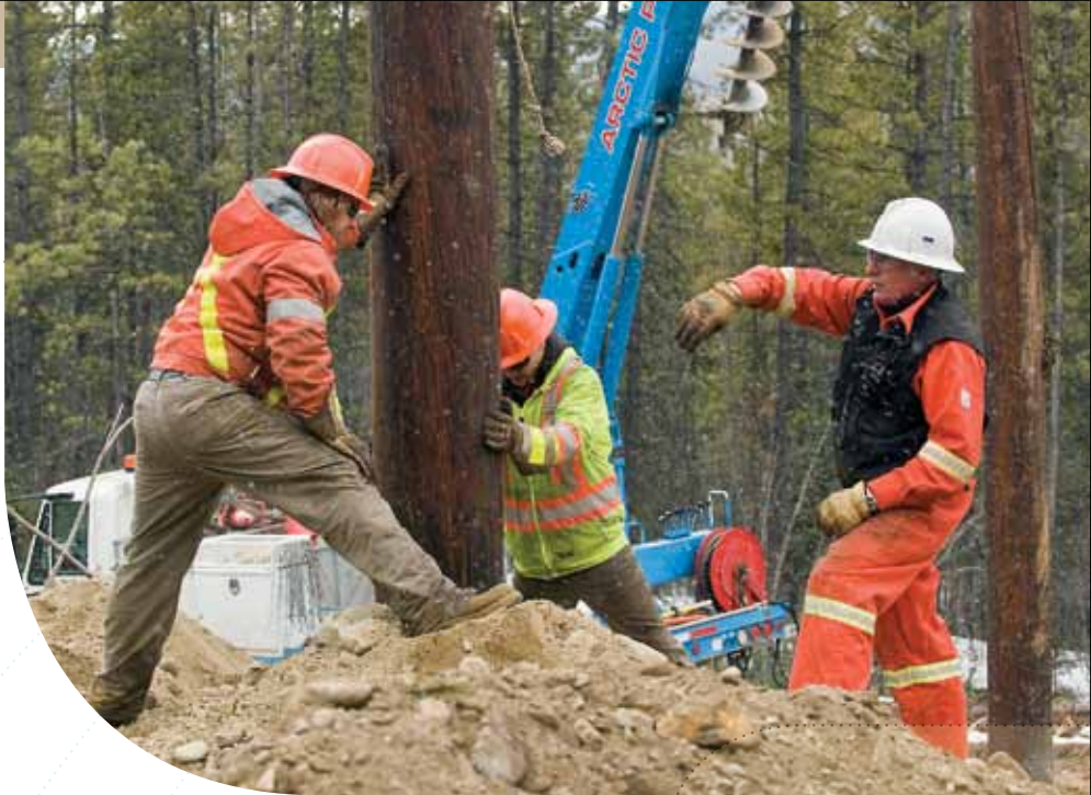
Setting poles on the Carmacks-Stewart line. Photo: www.archbould.com
