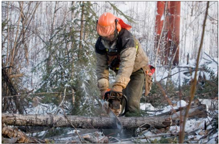
Clearing to make way for the transmission line. Photo: www.archbould.com
