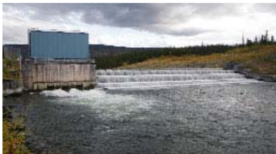
Wareham Dam. Photo: EDI Environmental Dynamics Inc.
