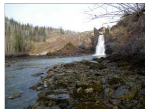
Wareham Lake spillway
