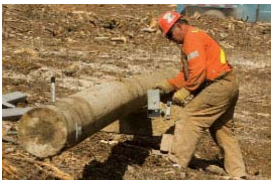
Assembling power poles for stage 1 of the Carmacks-Stewart line. Photo: www.archbould.com
