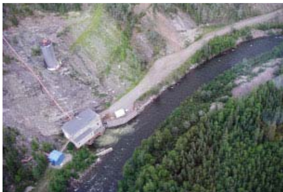
Aerial view of existing plant downstream from the Wareham Dam Spillway. Photo: Karl Scheifer
