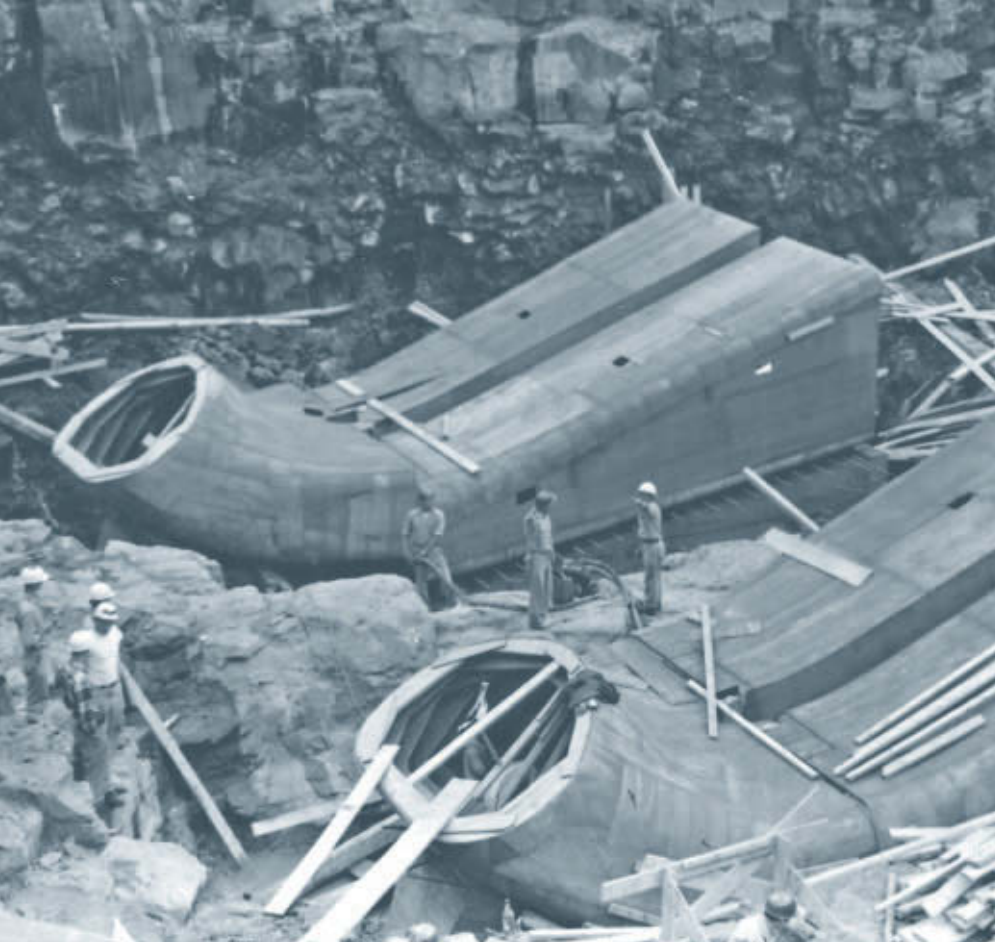
Draft tubes – dam construction c1957. PHOTO: Yukon Archives.
