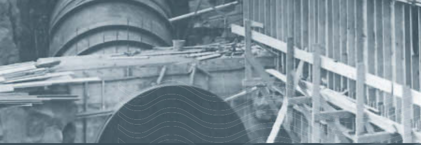
Left: Installing the penstock at the Whitehorse hydro facility. PHOTO: Yukon Archives
