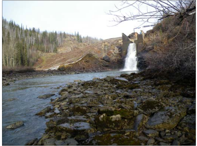
Wareham Lake spillway
