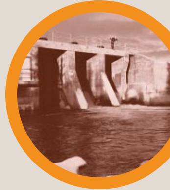
ONE OF THE CONTROL STRUCTURES AT THE AISHIHIK FACILITY
