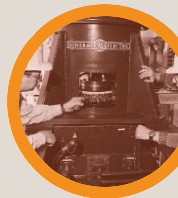
SENIOR POWERLINE TECHNICIAN CLINT KELLAND AND PLANT OPERATOR BOB GRINGAS IN THE MAYO PLANT
