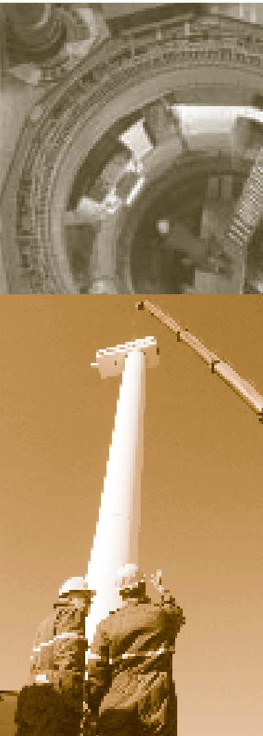
top: refurbishing one of the Whitehorse hydro turbines – Archbould Photography bottom: repairing the Vestas wind turbine on Haeckel Hill – Derek Crowe
