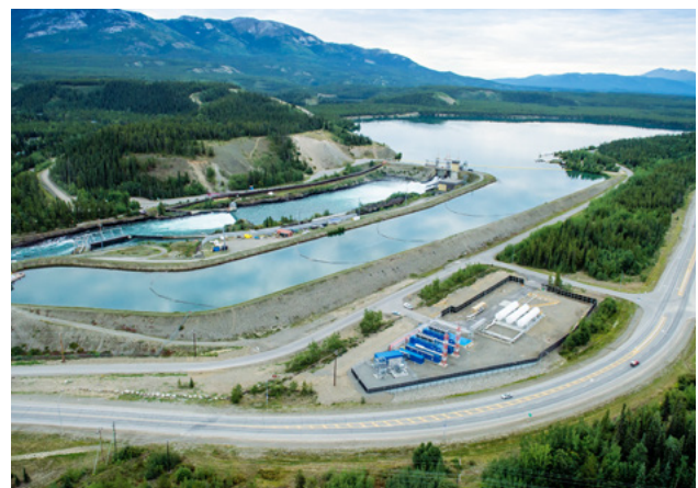
Aerial view of the Whitehorse Dam. Photo credit: Archbould Photography
