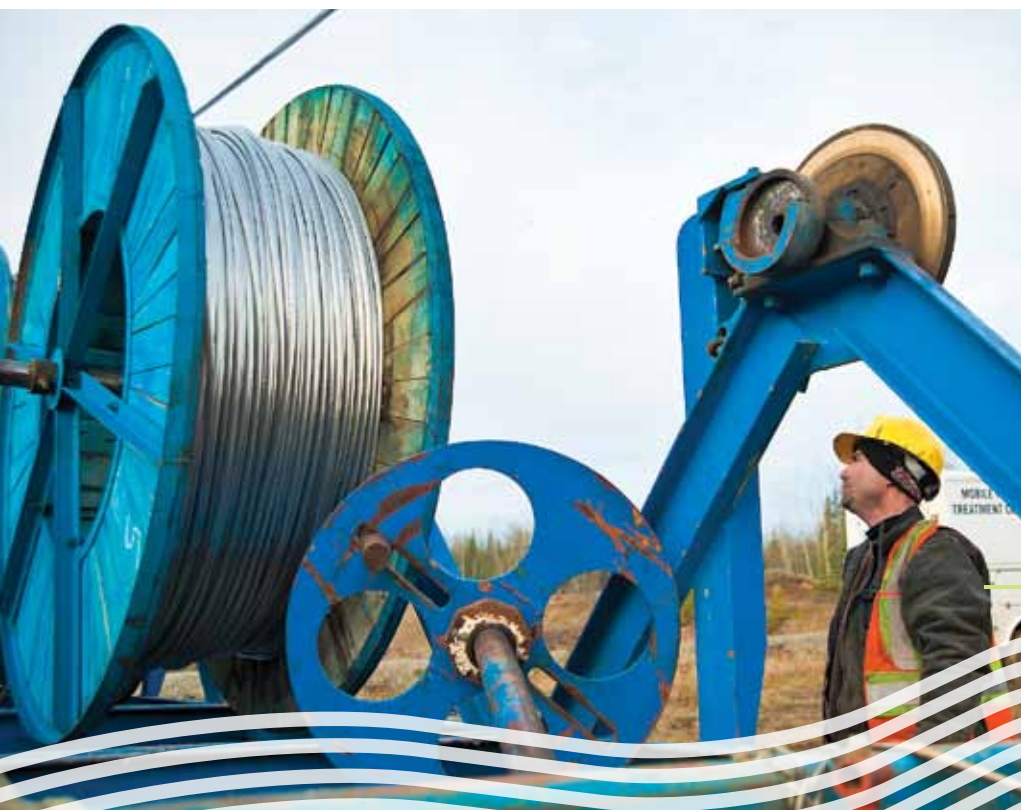
Stringing line for the Carmacks— Stewart Transmission Project Stage 2.
