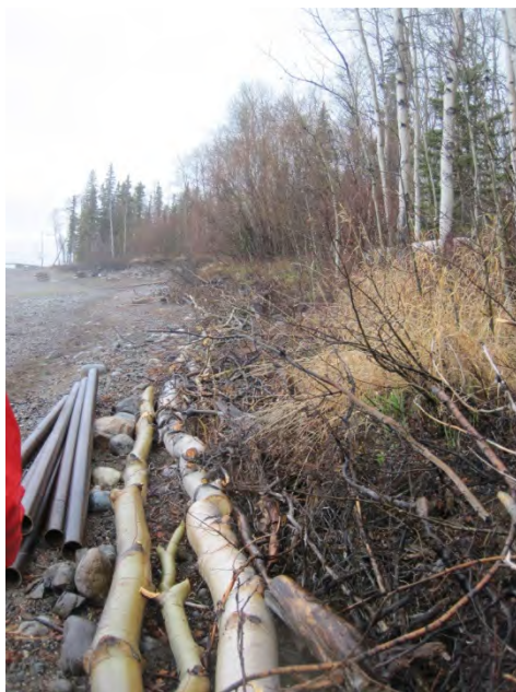
Photograph 6. View of erosion protection (logs) near Lot 79.
