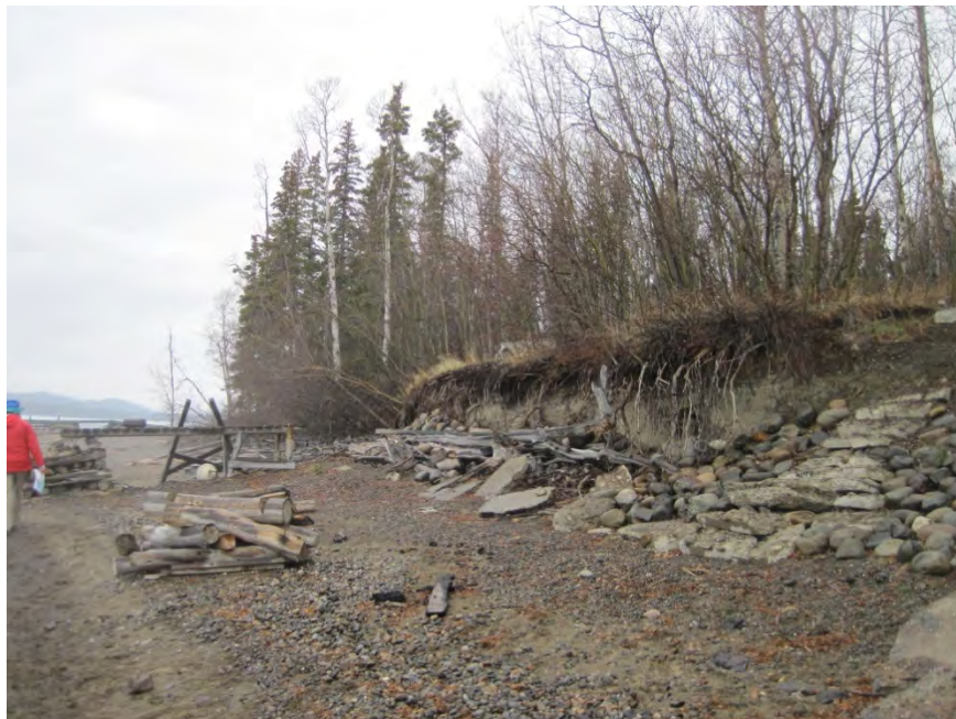
Photograph 10. View of erosion bluff near Lot 77 with some erosion protection (logs and boulders).
