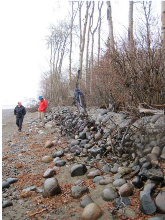
Photograph 9. View of flood and erosion protection (boulders and sandbags) near lot 83.
