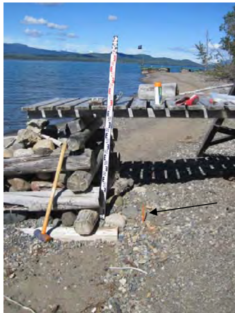
Photograph 2. Proposed FSL rebar installed (Lot 77)
