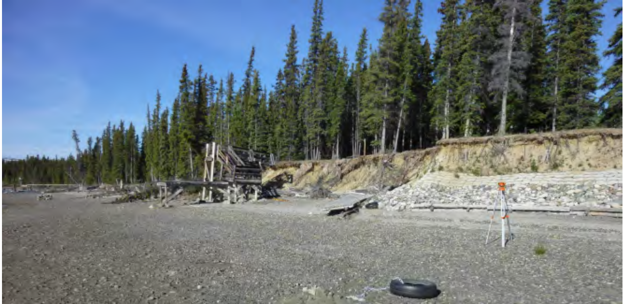
Photo 2 taken on beach in front of Lot 51, looking south, showing rock erosion control structure along bank in front of Lot 51 and eroding bank in front of Lots 52 and 53. Sand bags were placed during 2007 flood to control high water
