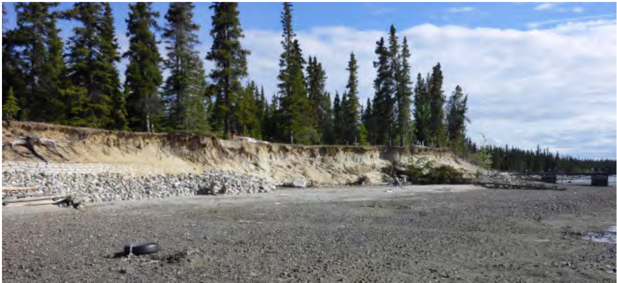
Photo 1 taken on beach in front of Lot 51, looking north, showing rock erosion control structure along bank in front of Lot 51 and eroding bank in front of Lots 40 and 49. Sand bags were placed during 2007 flood to control high water
