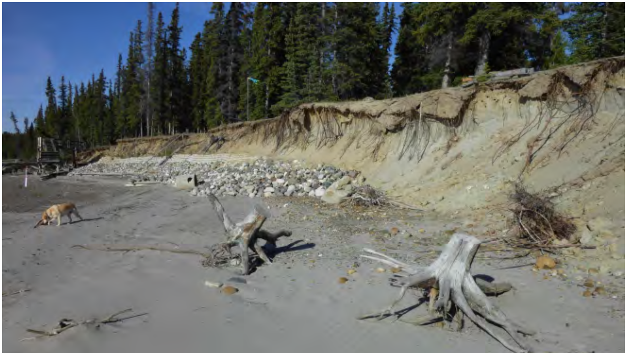
Photo 3 near toe of bank (OHWM) in front of Lot 50, looking south, showing rock erosion control structure along bank in front of Lot 51 and eroding bank in front of Lot 50.
