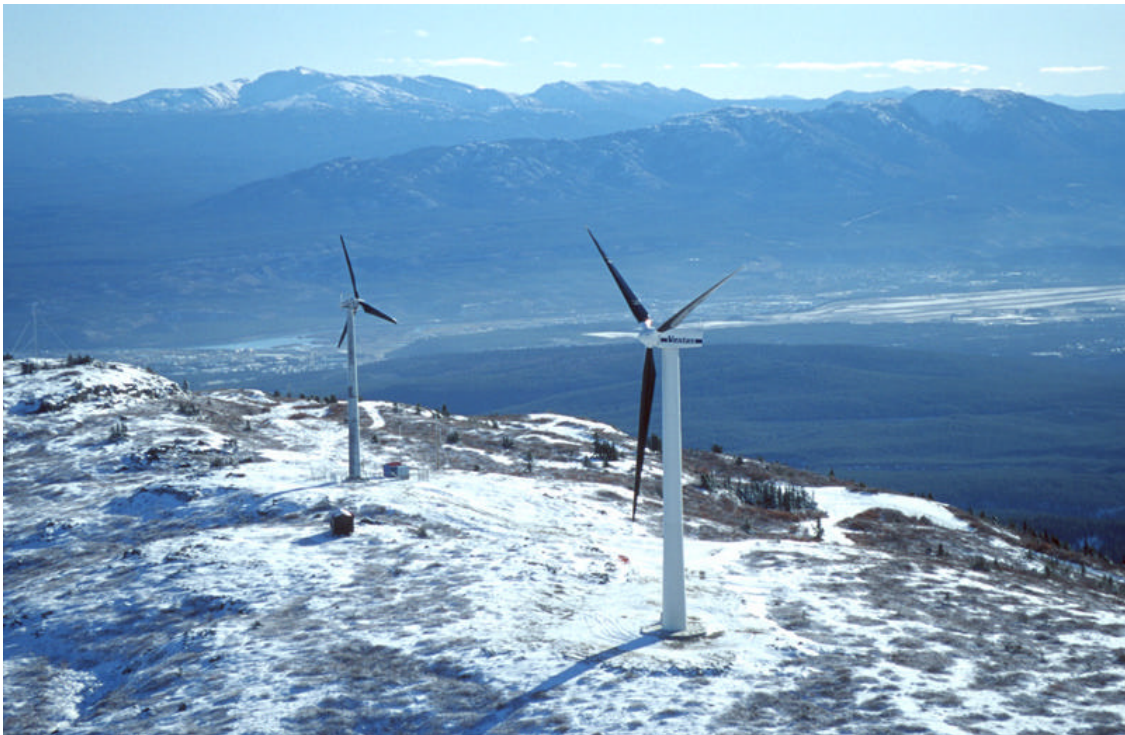
Photograph 10: both wind turbines in place
